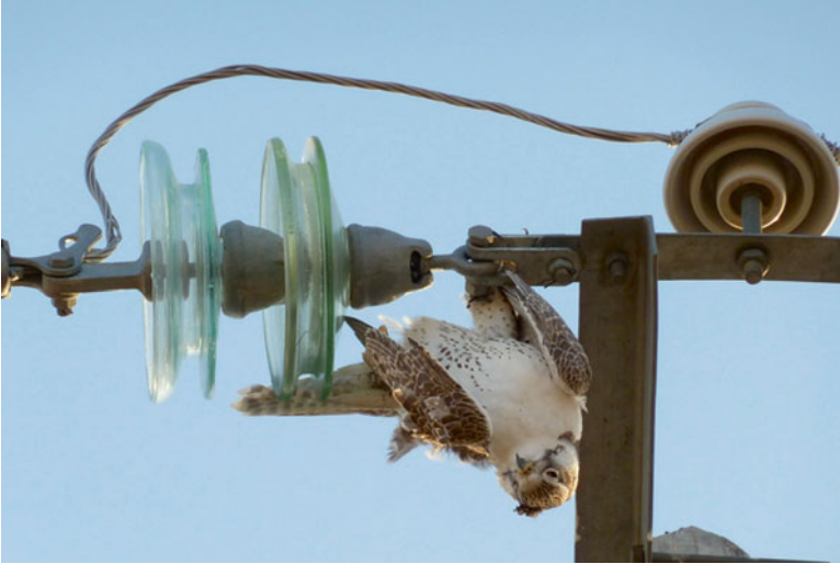
Fig. 4.4 Adult male Saker Falcon electrocuted at an anchor pole with a jump wire passing over the crossarm, Mongolia March 2012
